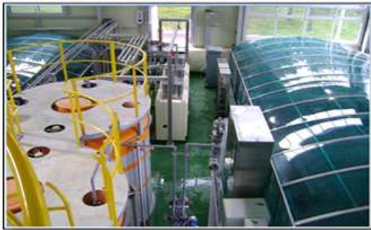
(a) Sealing of DOF by cover
