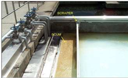
(b) Removing scum (floated flocs) by skimmer
